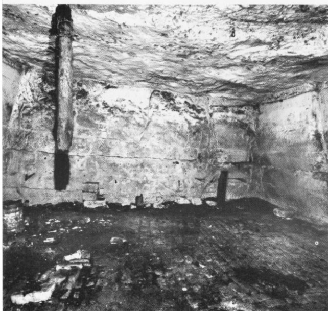
The interior of the underground stable. Note the cobbled floor to ease mucking out. Photo Nick Catford
